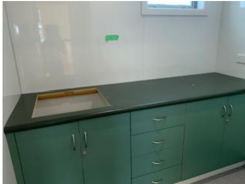
New Utility Room (utilising “old” kitchen cabinets)
